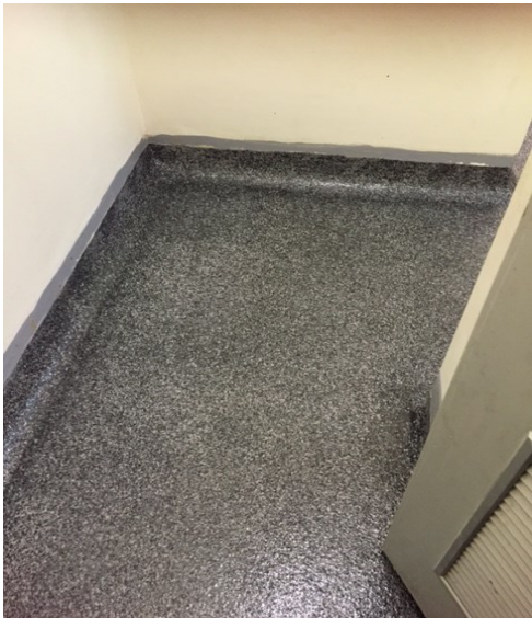
New toilet floor
